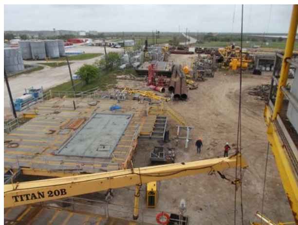
New Main Deck under construction.
