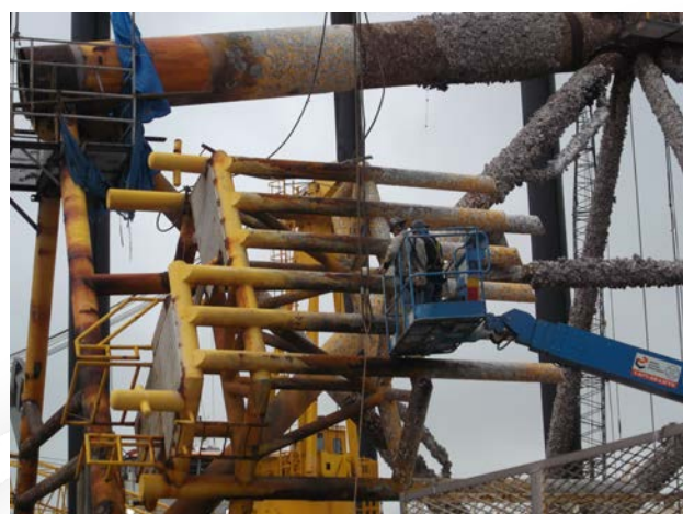
Tripod Refurbishment Underway.
