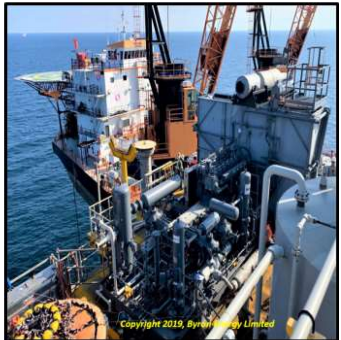
SM71 compressor upgrade construction spread
