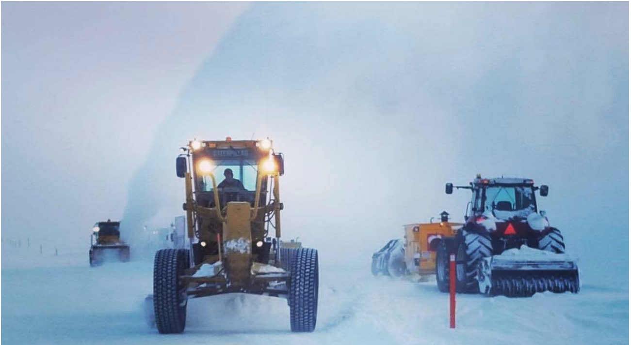
Figure 3 – Ice road construction.
